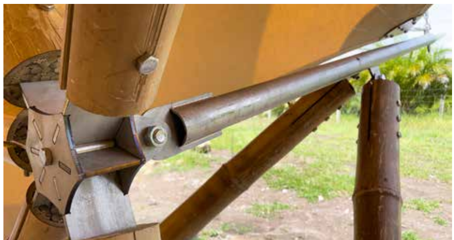
Bamboo joiner structure
