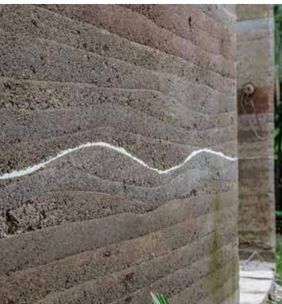
Close-up view of the wall using rammed earth construction, showing the striated and polychromatic layers of compacted earth.
