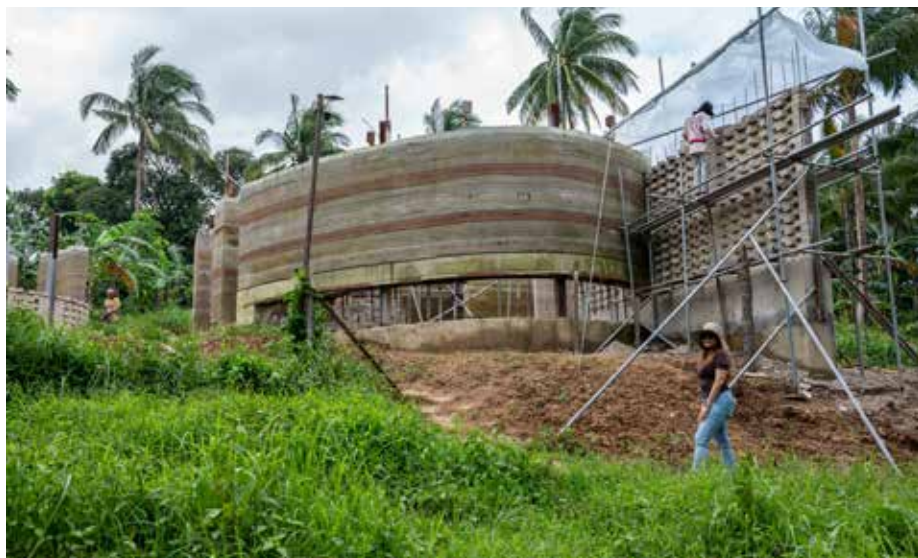
Left: Various wall systems used for the Sibol Farm Villa, including rammed earth and the Shear Key Interlocking System
