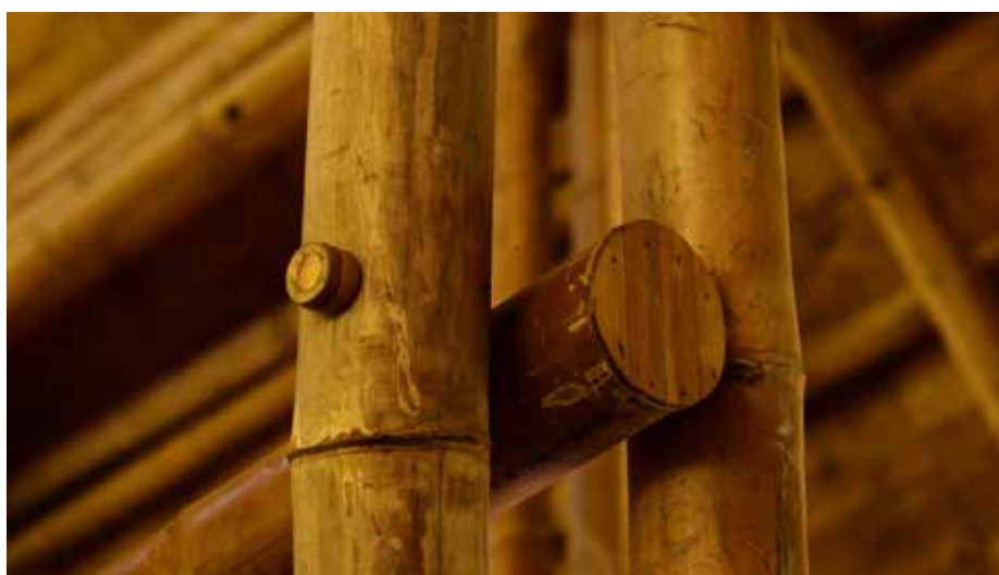
Connection details of bamboo joinery
